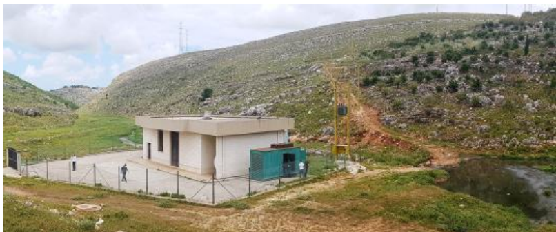
The pumping station and access road in En Nmairiye (Nabatieh), which CSP will rehabilitate under the wastewater management component.
