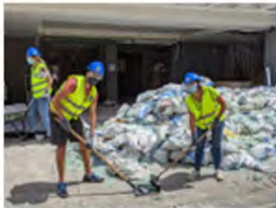
Photo credit: Community Support Program (CSP) ██████ shovel debris off the streets of an eastern Beirut neighborhoods damaged in the Beirut blast. They are on a team of workers being paid USD 20 per day by USAID’s CSP to remove rubble and debris from the city using a mix of heavy machinery and manual labor.
