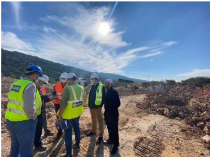
USAID/CSP and stakeholder visit to discuss the technical implementation of its solar activities in Hasbaiya on the land rented by the municipality to facilitate implementation – South Lebanon
