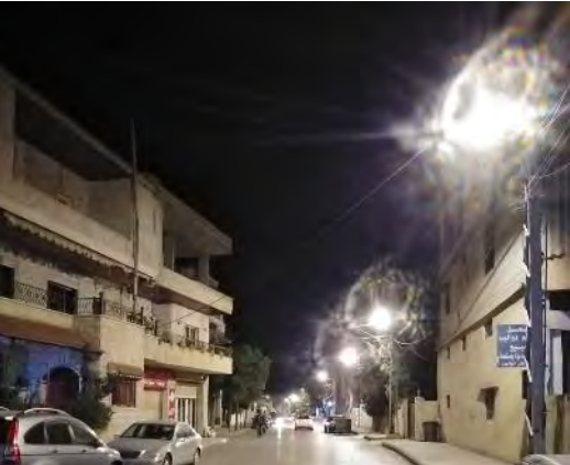
Photo showing the improved streetlighting conditions following CSP's interventions in El Marj (Beqaa)
