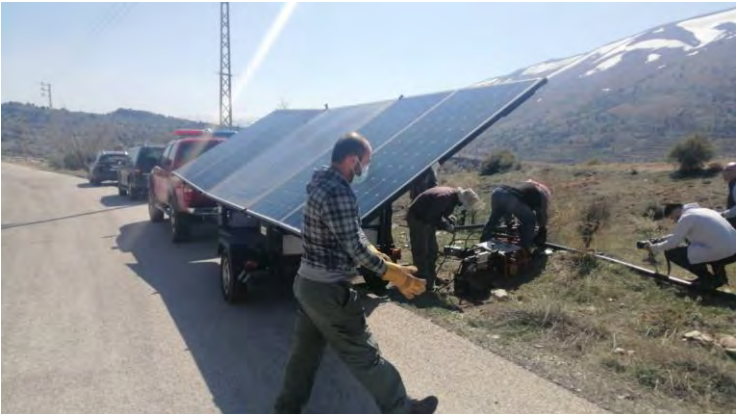
Ainata el Arz farmers utilize CSP’s provided solar welding machine to repair irrigation pipes
