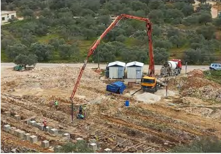
USAID/CSP ongoing works in Hasbaiya to supply and install on-grid solar farms
