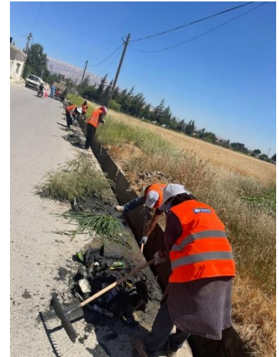
LIW being carried out in Qabb Elias
