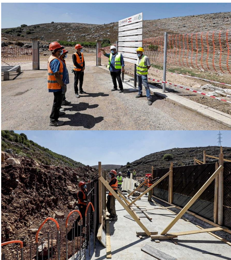
Ongoing implementation works in Nmaiye Pumping Station
