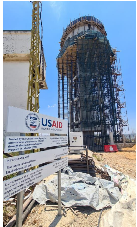
Progress on construction of the water tower in Jinsnaya, South Lebanon
