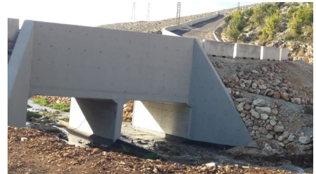
Constructed road to facilitate access to the Nmairiye wastewater pumping station
