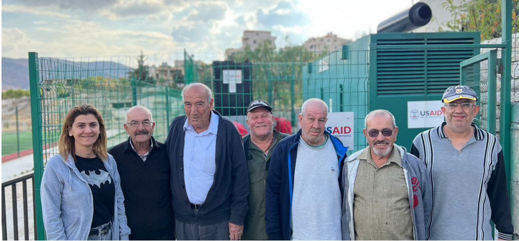
Municipal members and residents of Deir el Ghazal in front of USAID/CSP's provided generator which is enabling access to essential services for more than 1,750 residents
