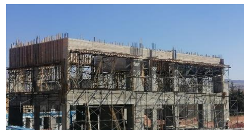
Progress on new dewatering building in Aaitanit
