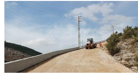
Ongoing works on the access road to Nmairiye Pumping Station.
