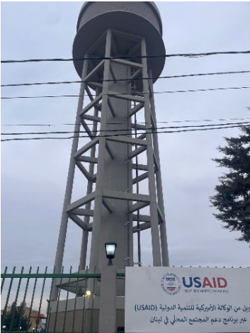
Progress on construction of the elevated water tank in Talia at 95%
