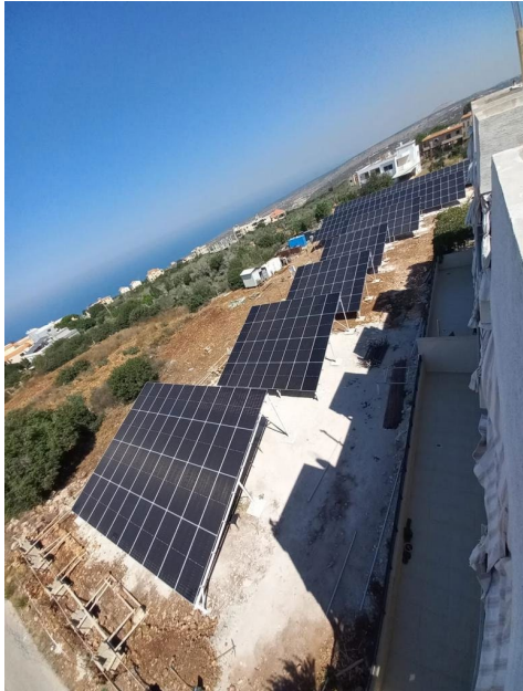
Site in Aalma ech Chaab, where CSP is installing a solar farm to hybridize the town's electricity system
