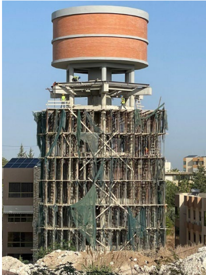
Progress on the construction of the elevated water tank in Bqasta, before and after the removal of the scaffolding
