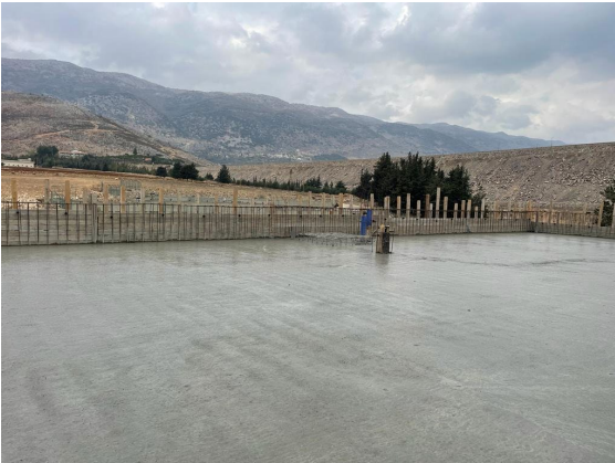
Concrete pouring of the dewatering building’s roof slab
