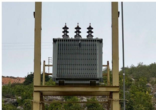
Installation of the new 450 KVA transformer
