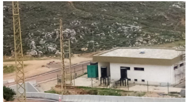
The wastewater pumping station building, the box culvert and the refurbished antiwater hammer vessels at Nmairiye pumping station
