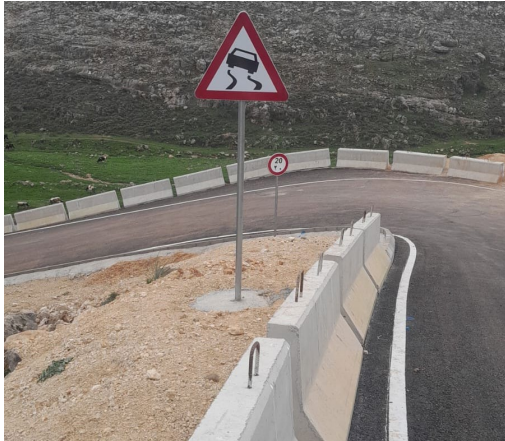
Installation of signpost along the Nmaiye access road
