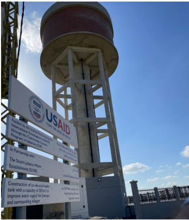
Progress on construction of the elevated water tank in Jinsnaya
