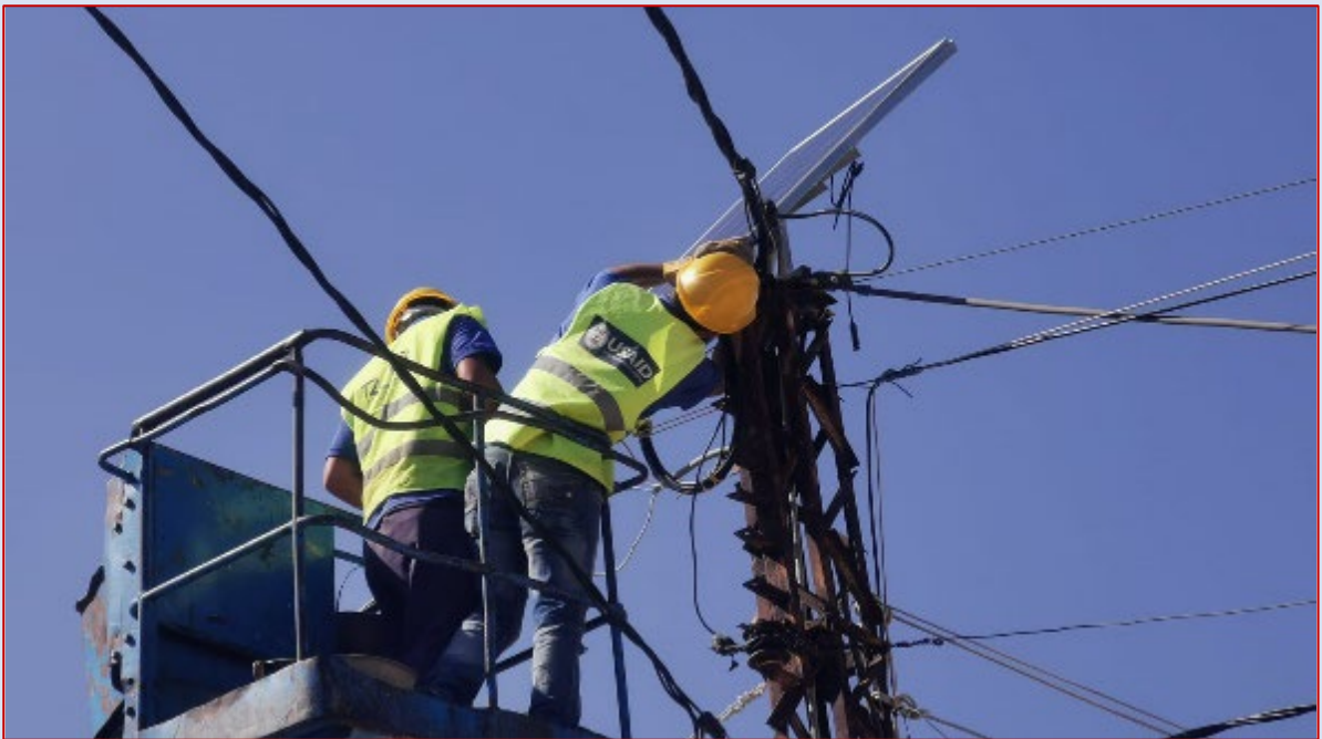
CSP installs solar streetlights in Kfar Jarra, South Lebanon
