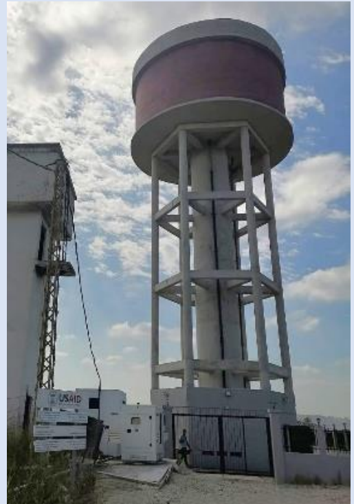
The CSP-constructed 300 m 3 water tank in Jinsnaya, South Lebanon – Dec , 2023
